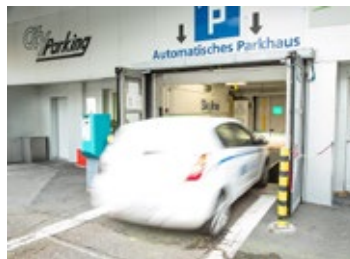
City Parking Schaffhausen, Switzerland The only public Automated Parking System in Switzerland
